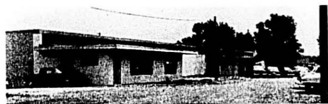
THE NEW ONE-STORY BUILDING housing King Midas Flour warehouses and the Galioto Brothers macaroni plant.
