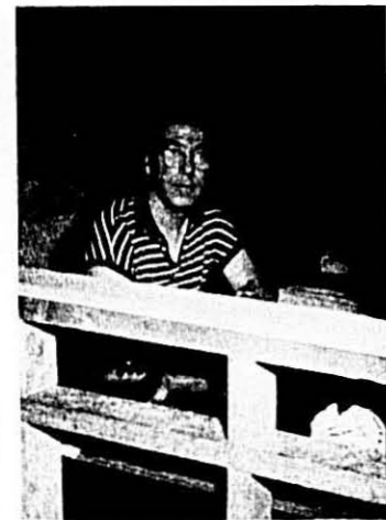
JOHN GALIOTO does his paper work while construction goes on.
